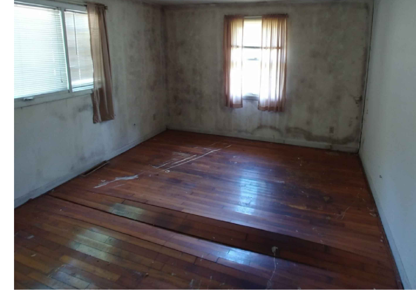
6 BUCKLED WOOD FLOOR
