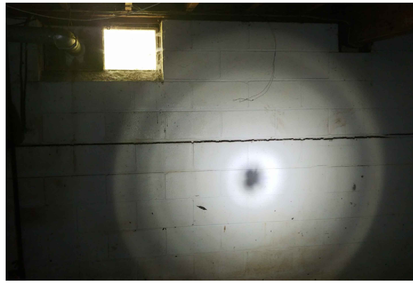
2 FOUNDATION WALL CRACK / MOVEMENT
