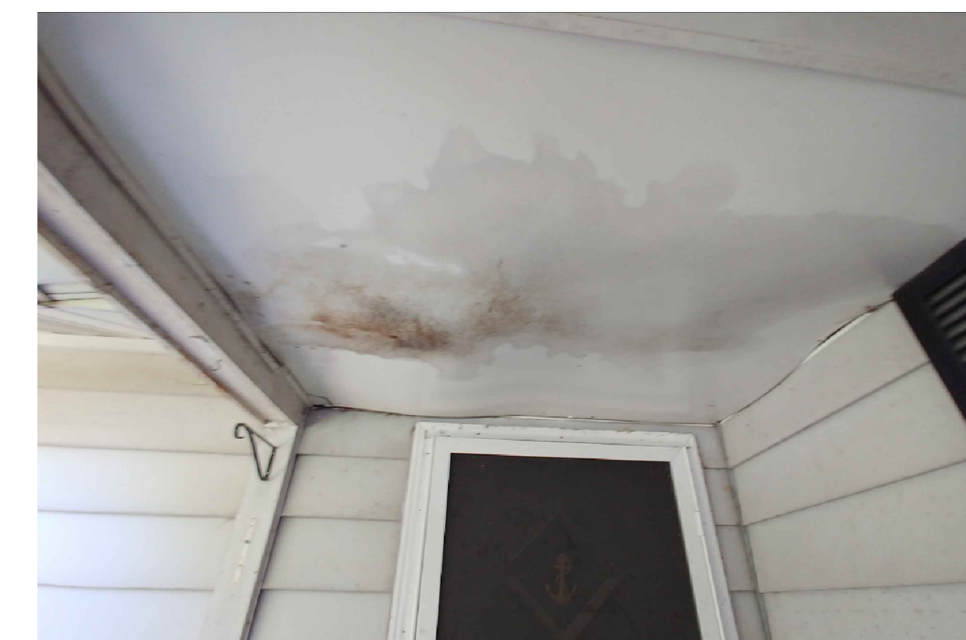
11 FRONT PORCH CEILING
